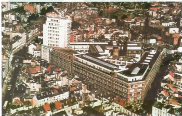
Headquarters of Bell Telephone Mfg Co, Antwerp Belgium, and birthplace of the Metacocta 10 C system.
